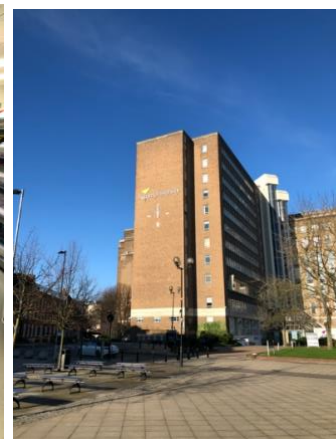
Main Building Aston University
